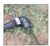
Pull the cable through the elbow, and screw the 3/4" 90° M-F elbow to the poly riser.
