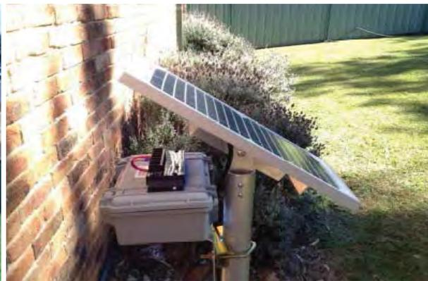
Photo 8: Optional Battery Pack & Regulator fitted.
